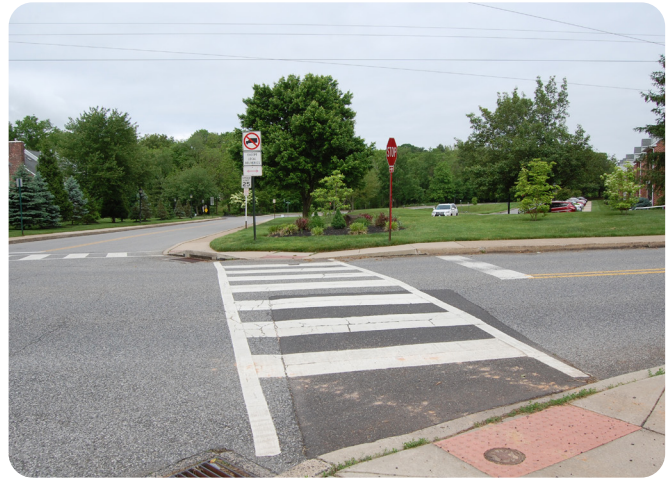
Figure 11. Crosswalk at Park and Third Avenues
